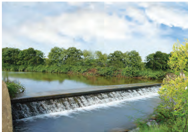
2.3.9 Concrete cement stream check dams
