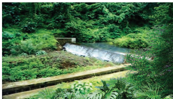
2.3.10 Diversion check dam
